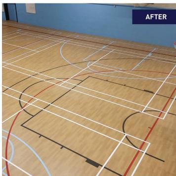
"The Isolsport underlay also supplied by Gerflor, enabled us to lay the Taraflex<sup>®</sup> Multi-Use directly over the existing concrete floor, this was a real benefit as the project was on a very tight schedule, due to the hall being required for exams."
