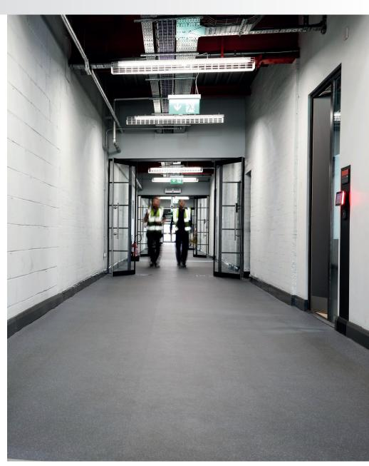
We chose the Gerflor Attraction® floor tile down to the sub floor issues which meant we had to rule out many alternative conventional flooring methods, thus, we had to find a solution that was not bonded to the existing surface.
