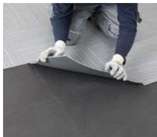
Apply planks or tiles
