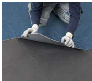
Apply planks or tiles
