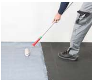
Installation with tackifier
