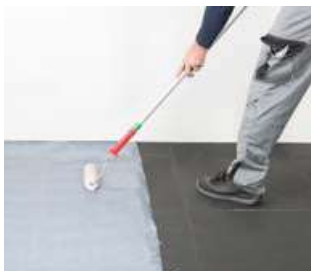
Installation with tackifier
