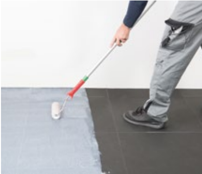
Application of the pressure sensitive adhesive
