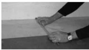
Place the sheet to cut on the sheet beside making sure it is correctly aligned (edges must be parallel).
