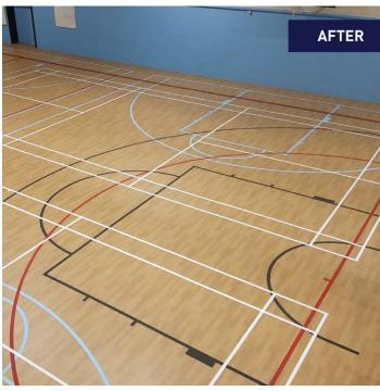
"The Isolsport underlay also supplied by Gerflor, enabled us to lay the Taraflex® Multi-Use directly over the existing concrete floor, this was a real benefit as the project was on a very tight schedule, due to the hall being required for exams."
